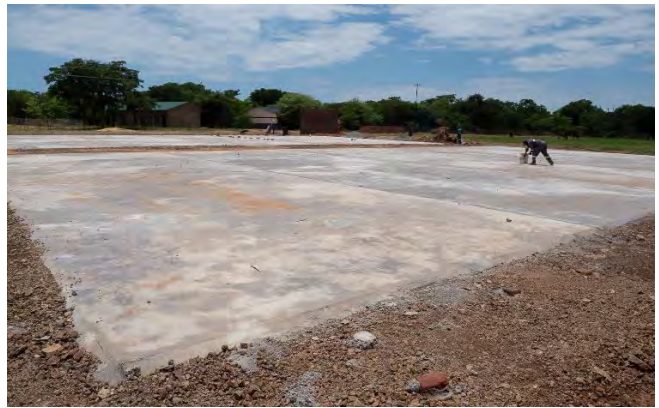
New sports facilities being constructed
